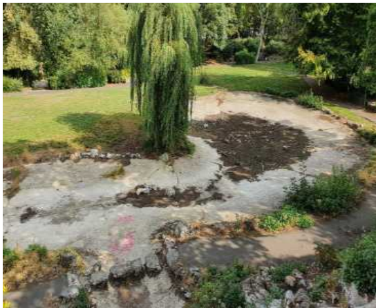
Rockliffe Gdns – Redundant pond, restore create wildlife pond
