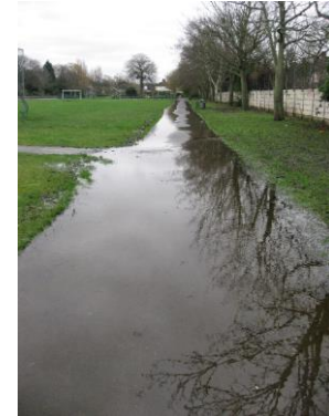
Plumstead Gdns - Flooding survey and resolve
