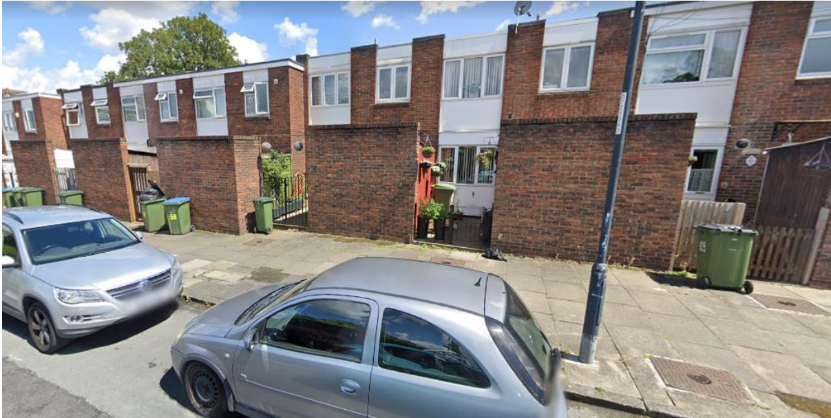
Figure 8 Existing Properties on Palmerston Crescent
